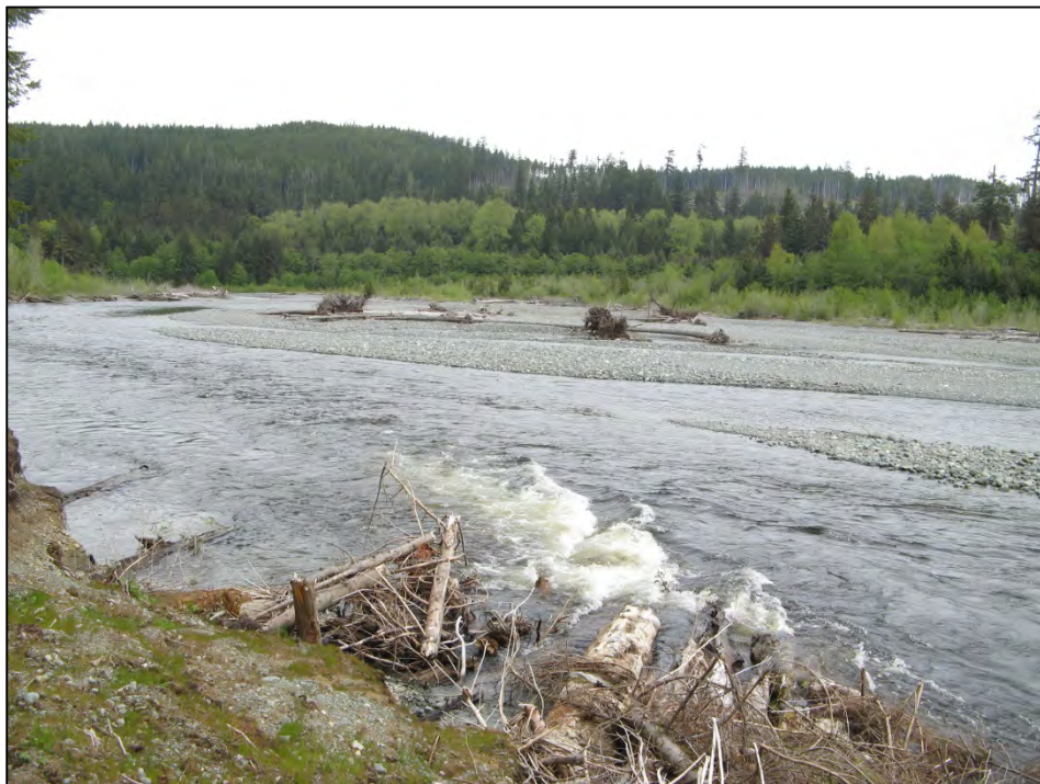
Photo 9. Large woody debris revetments installed on an eroding left bank of the Eve River.
