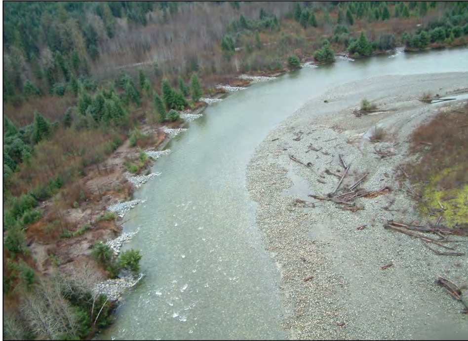
Photo 8. Rock groynes constructed on an eroding left bank in the Phillips River.
