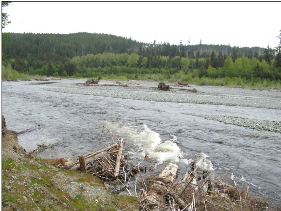
Photo 7. Large woody debris revetments installed on an eroding left bank of the Eve River.
